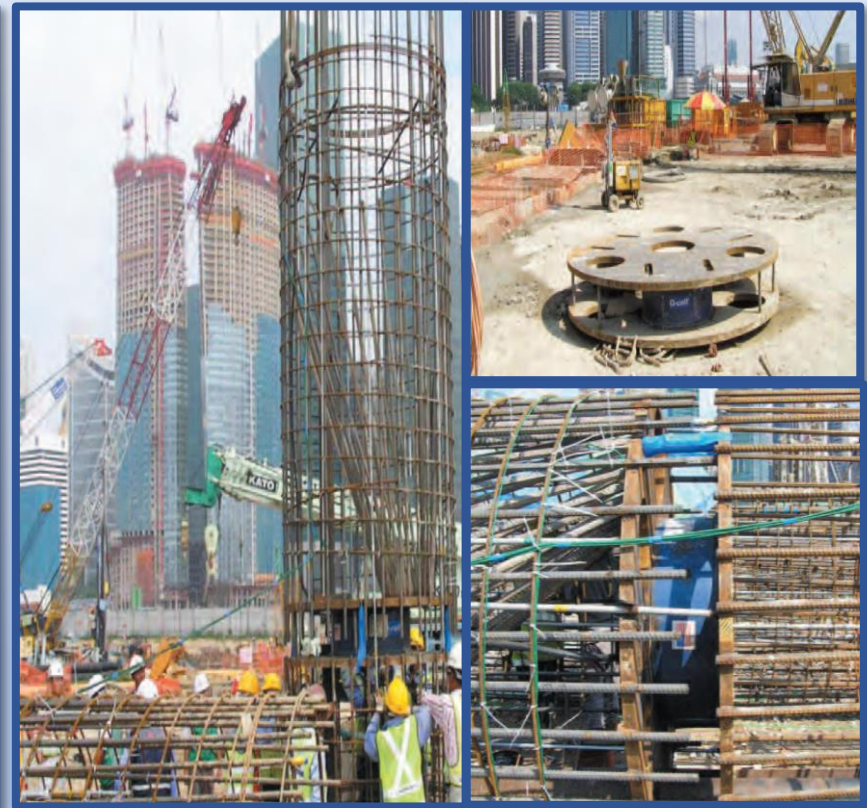
O-Cell implementation in Marine Bay Sands project (Foundation Drilling, 2012)
